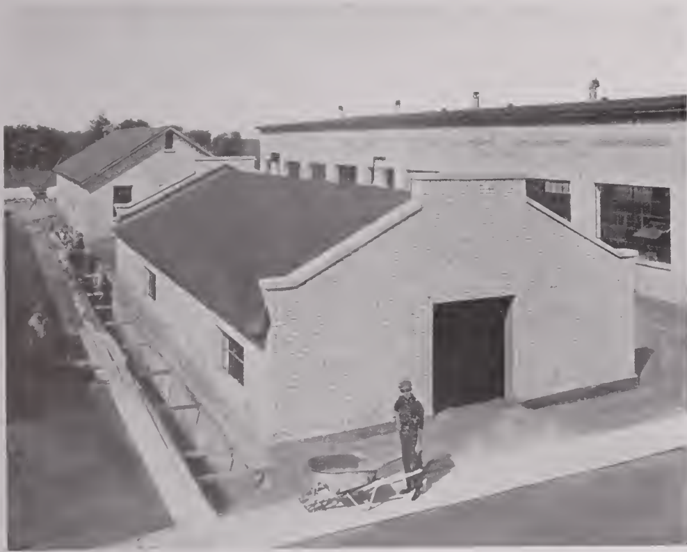
THE OIL STORAGE BUILDING
